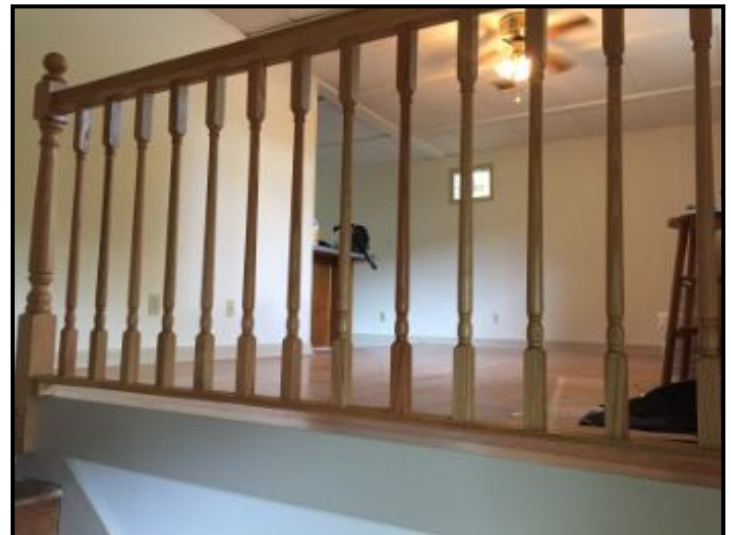
Look to be in good condition
