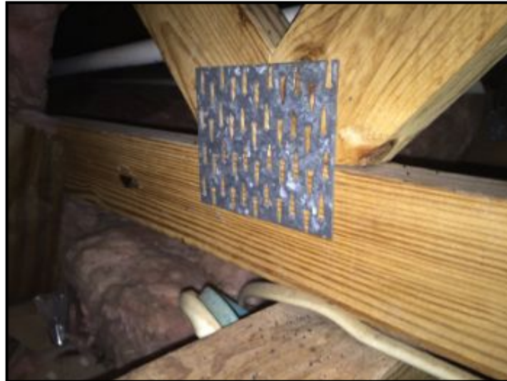
Metal gusset plate used to hold beams to joists.
