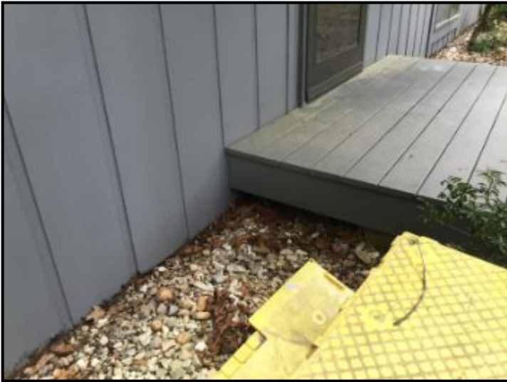
Front porch looks to be almost new condition
