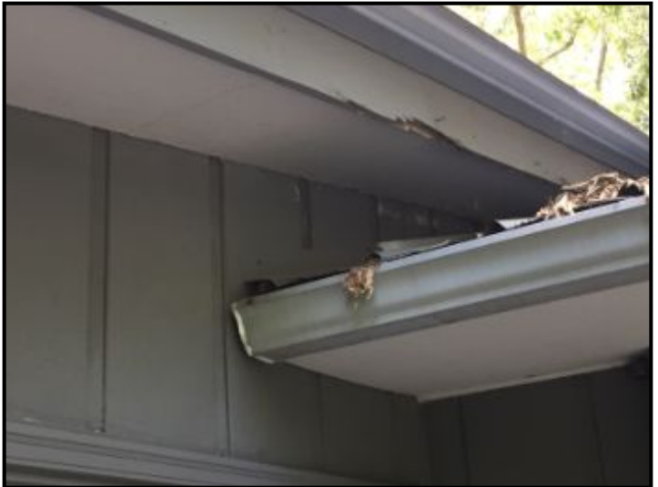
Eave and fascia look good - note missing light bulb Some chipping damage on this fascia board - does not look like water damage
