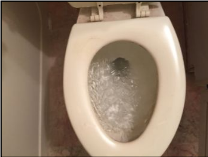
All toilets worked at time of inspection
