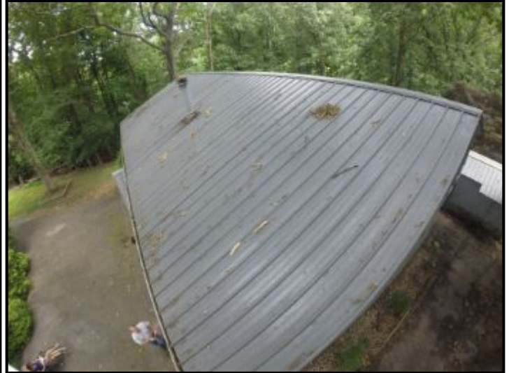
Overall condition of roof looks good
