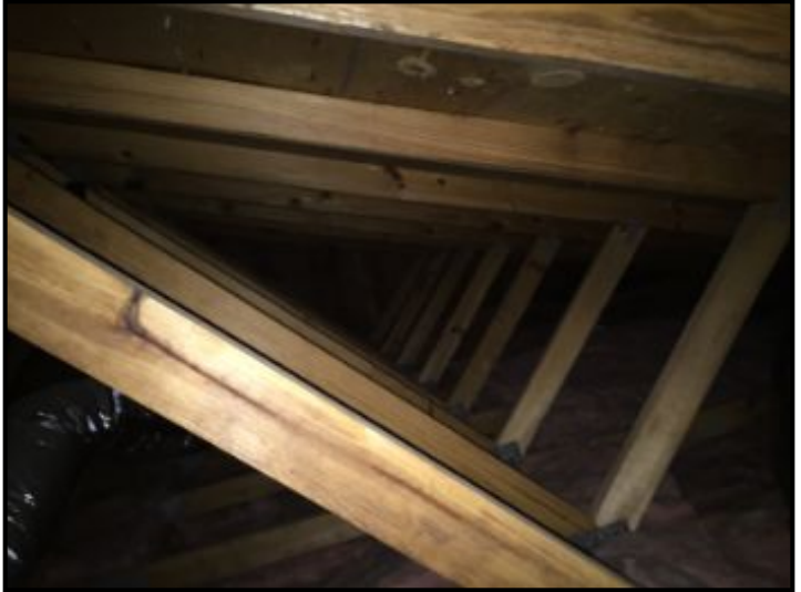
Wood supports look good with no defects noted
