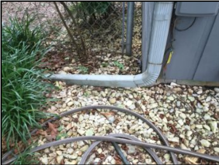
Down spouts appear to be in good working order.
