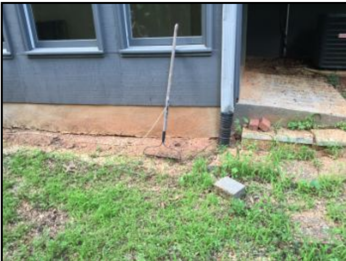
Gutter going into drain pipe away from house
