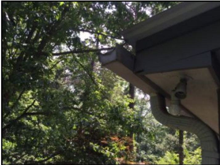
Eave and fascia look good - note missing light bulb Some chipping damage on this fascia board - does not look like water damage
