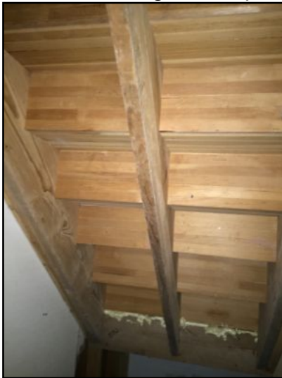
Underneath stair - structure looks good - no defects noted
