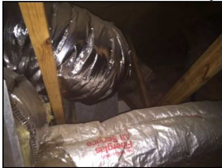
Ductwork condition looks good in attic
