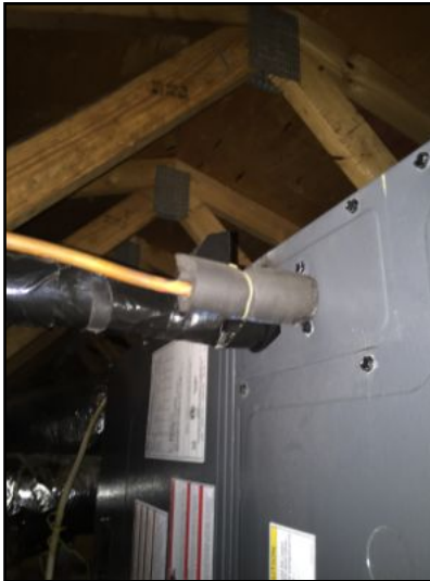
Heater in attic appears to be in good condition
