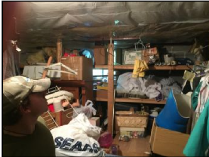
Extra room still has a lot of personal items in room - note plastic covering ceiling.
