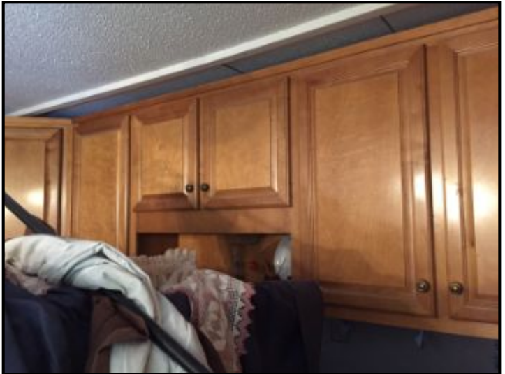
Cabinets look good, note clutter/bedroom furniture occupying kitchen area
