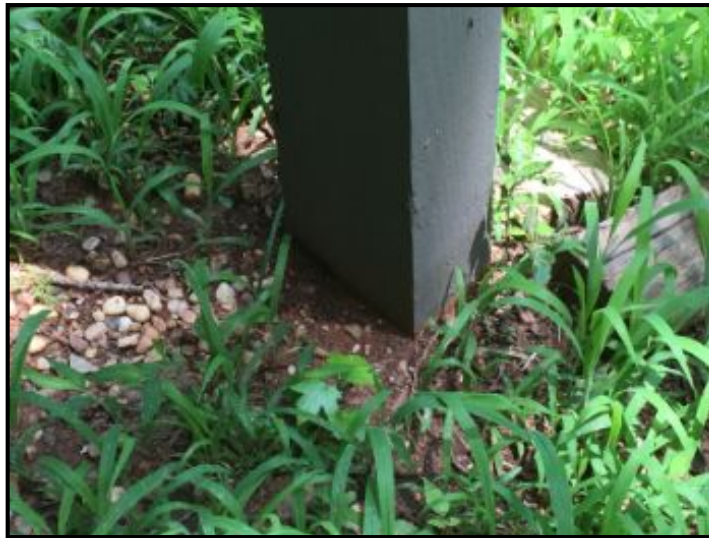
Porch base beams in good condition
