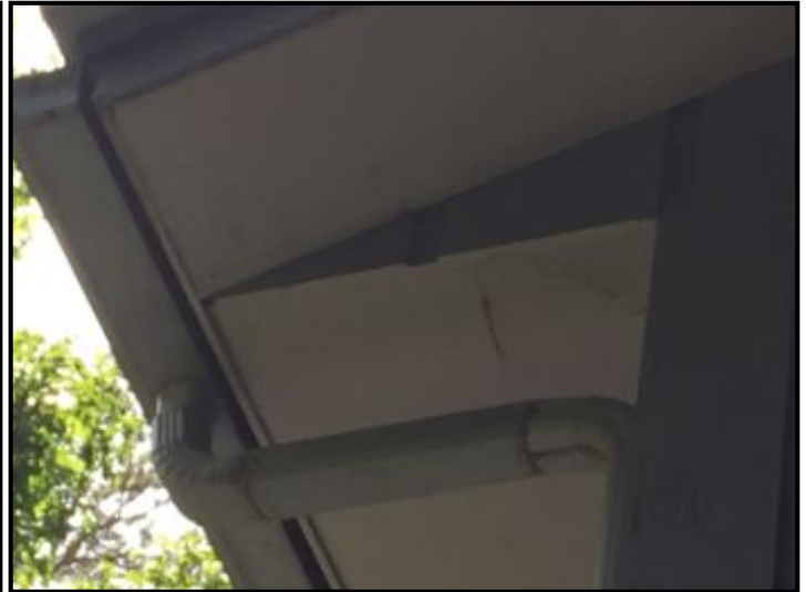
Eaves and facia in good shape - note spider web - not damage.
