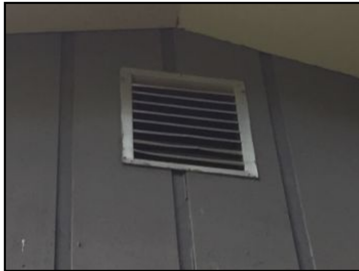
Gable vent at end of house - attic was cool
