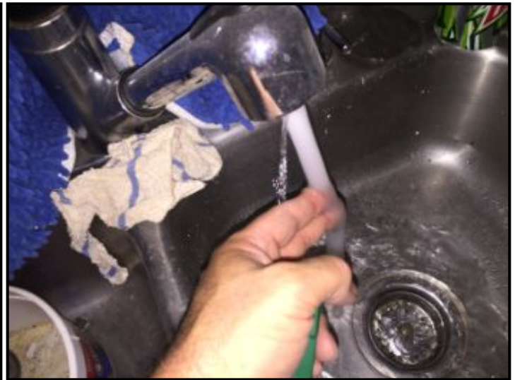
Warm water noted during inspection - possible water heater had not warmed up completely during inspection
