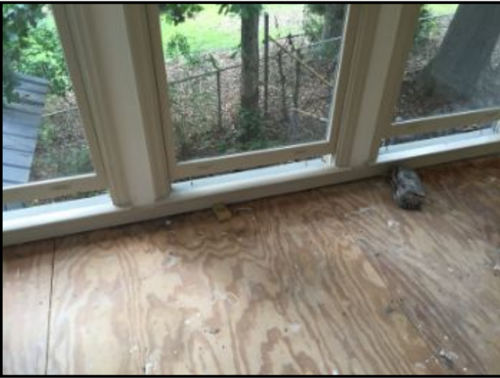
Windows functioned properly
