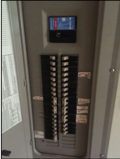
Main breaker worked properly at time of inspection
