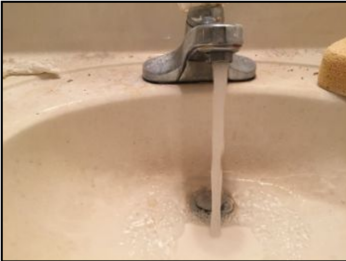
Sinks worked at time of inspection
