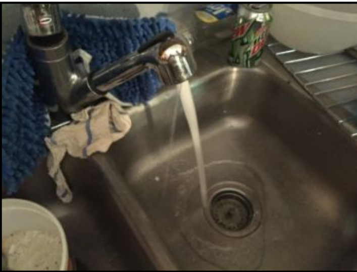
Kitchen sink seen working at time of inspection
