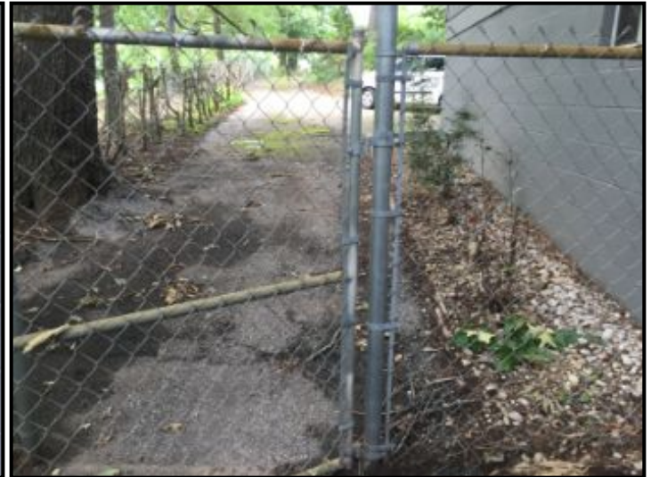
Both gate doors functioned properly at time of inspection
