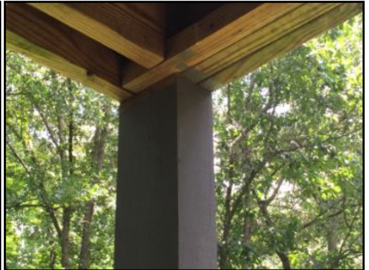
Structure supports on porch seem to be in good condition
