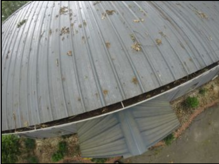
Roof condition looks good - gutters need cleaning
