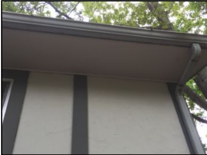
Eaves and facia boards look to be in good shape.
